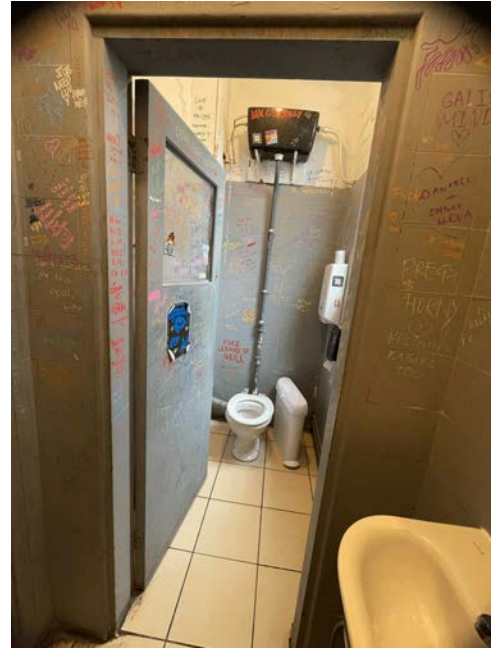
Cubicle door 27 inches wide. Push to open.
