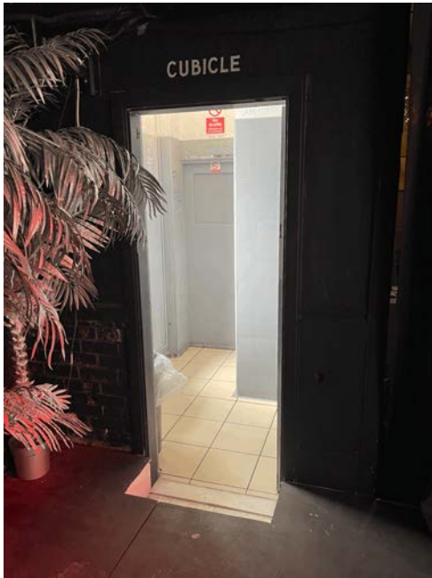
29 inches wide. 8.5 inch step. Push to open.
