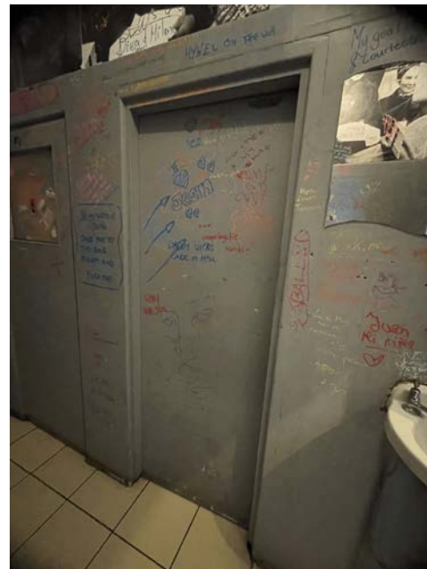
Cubicle door 27 inches wide. Push to open
