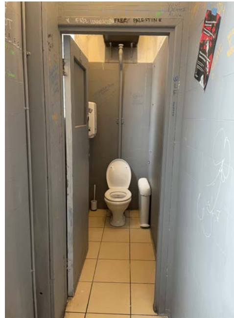
Cubicle door 27 inches wide. Push to open
